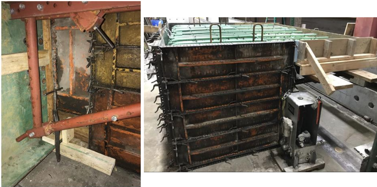
Figure 4.31 GRBC integral diaphragm formwork.
