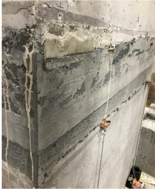
Figure 4.23 Completed UHPC joint showing the multiple layers of material.
