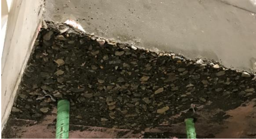
Figure 4.17 UHPC integral diaphragm exposed aggregate finish.
