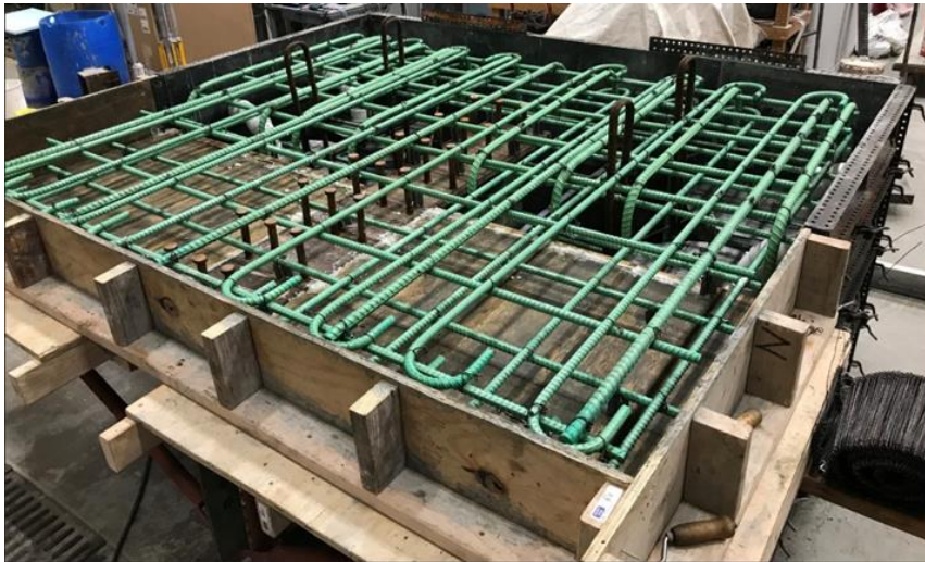
Figure 4.51 Pile coupler reinforcement cage.
