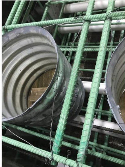
Figure 4.41 Metal wire holding CMPs in designed locations.
