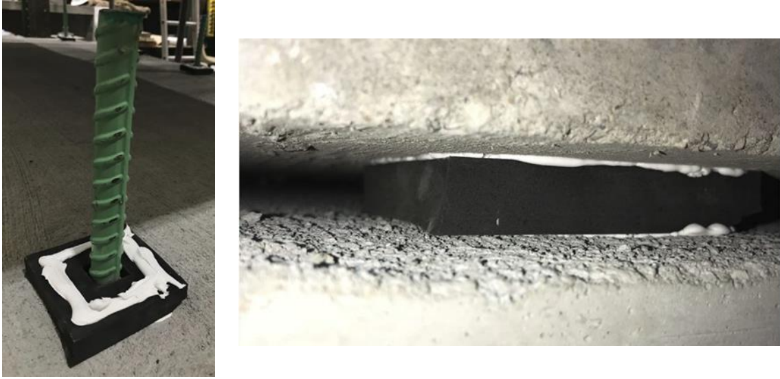
Figure 4.35 GRBC 3/4 in. neoprene pad and silicone seal.
