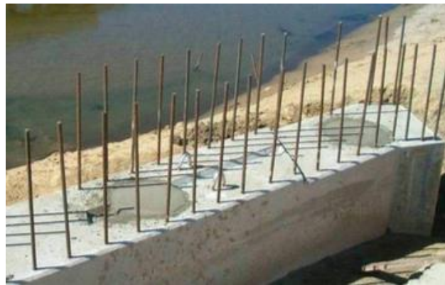
Figure 2.22 Finished abutment cap with CMP voids filled. (Wipf, Klaiber, & Hockerman, 2009)
