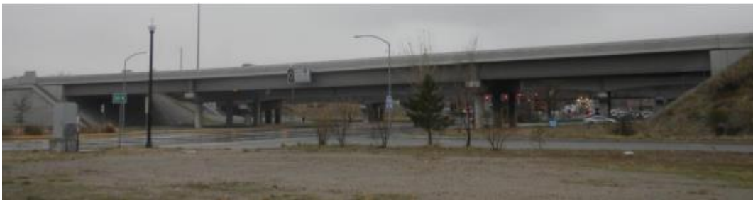
Figure 2.64 Photograph of 400 South Street Bridge in elevation view. (Huffaker, 2013)
