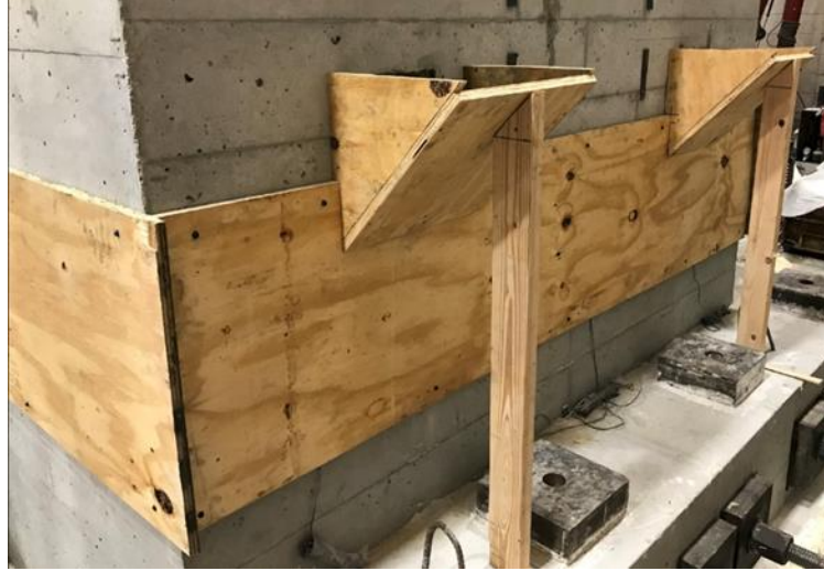
Figure 4.21 Rear face joint formwork with chimneys.
