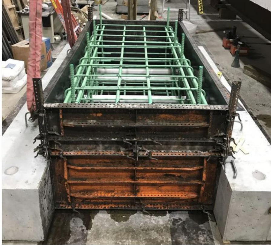
Figure 4.25 GRBC pile cap formwork.
