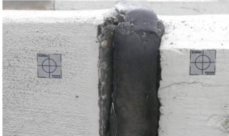
Figure 2.66 Survey targets at approach slab. (Huffaker, 2013)
