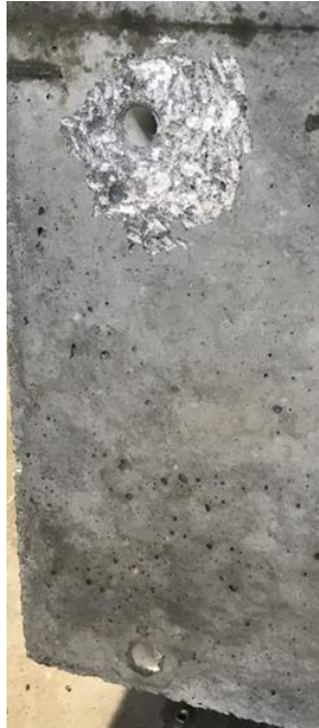
Figure 4.33 GRBC grout sleeve ports located post concrete casting.
