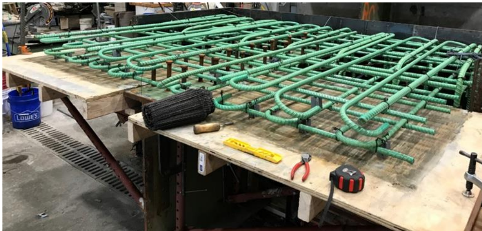
Figure 4.11 UHPC integral diaphragm reinforcement cage completed.
