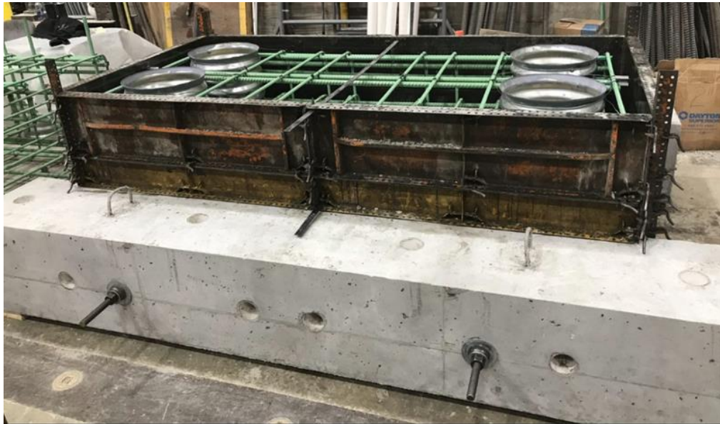
Figure 4.43 Pile coupler pile cap formwork.
