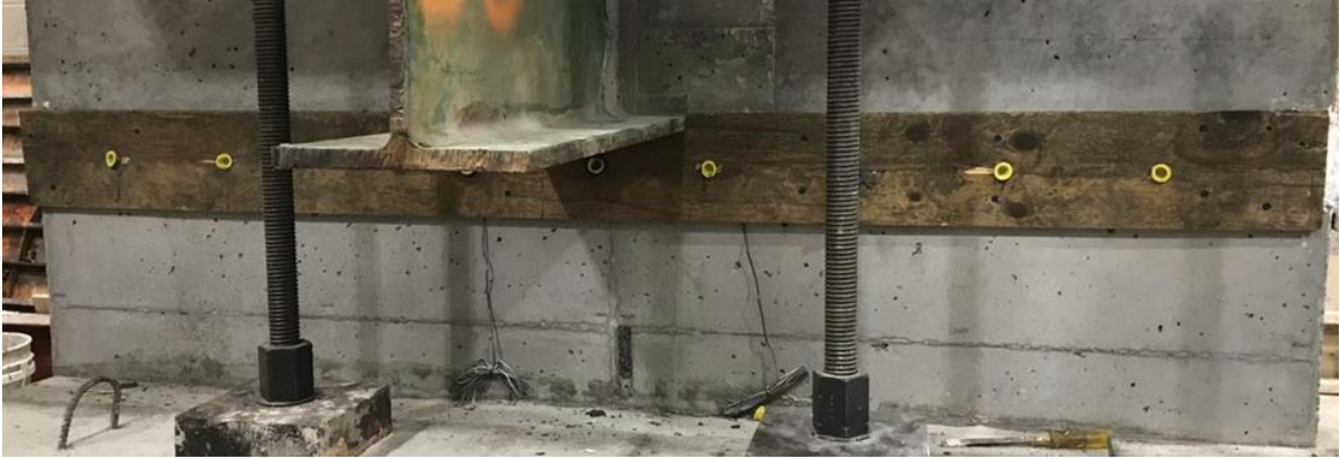
Figure 4.37 GRBC grout bed completed.
