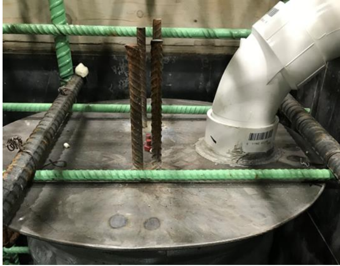
Figure 4.50 CMP “locking” reinforcing steel bar.
