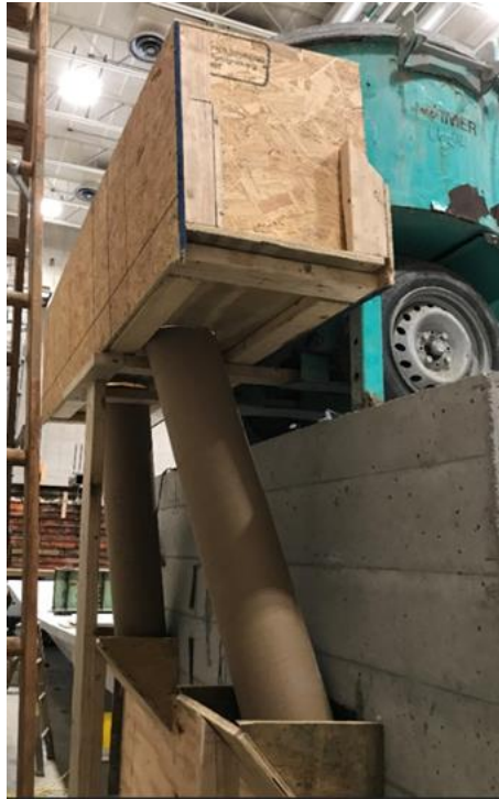
Figure 4.22 Spout and chimney system for installation of UHPC material.
