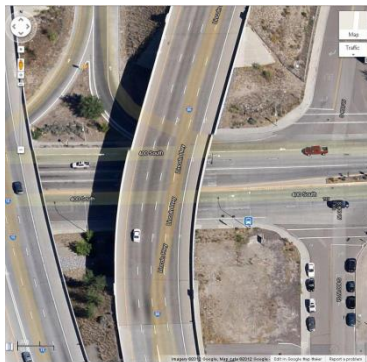
Figure 2.63 Aerial view of the 400 South Street Bridge. (Huffaker, 2013)
