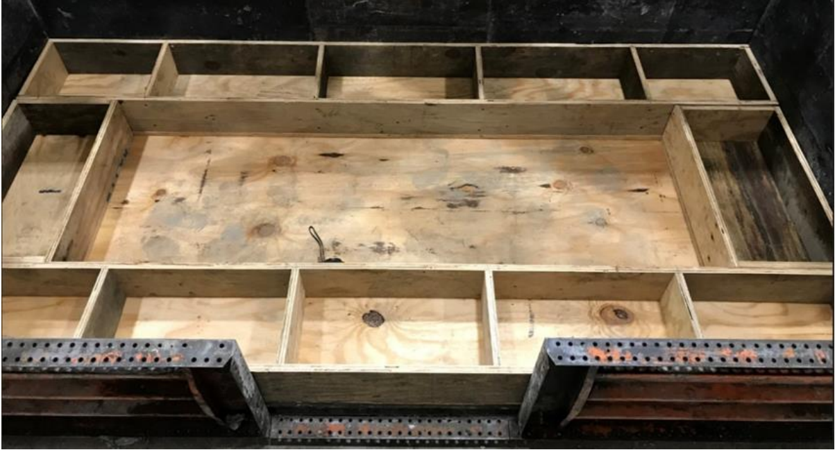
Figure 4.7 UHPC integral diaphragm formwork top view of diaphragms.
