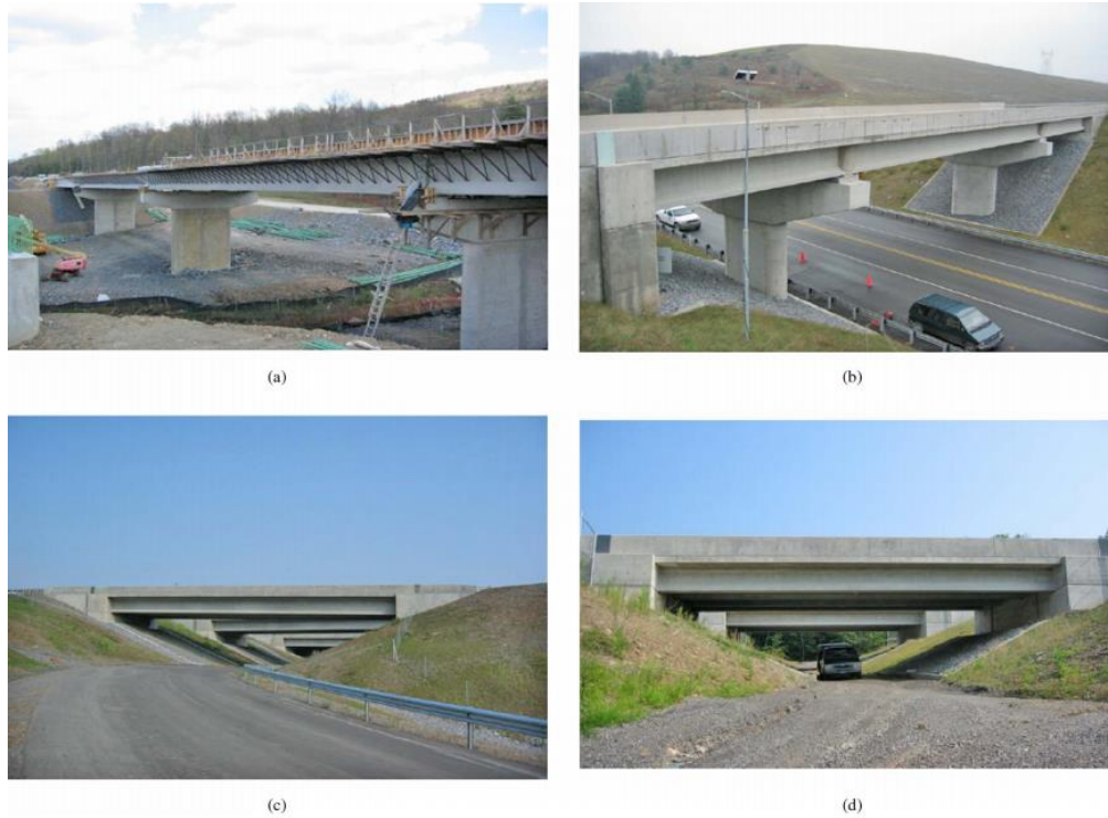
Figure 2.62 Instrumented bridges. (a) Bridge 109; (b) Bridge 203; (c) Bridge 211; (d) Bridge 222 (Kim & Laman, 2012)
