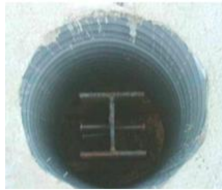
Figure 2.19 Abutment cap final position (left) H-pile in CMP void (right). (Wipf, Klaiber, & Hockerman, 2009)
