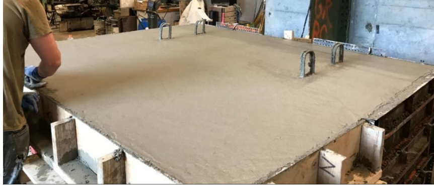
Figure 4.15 UHPC integral diaphragm cast in concrete.
