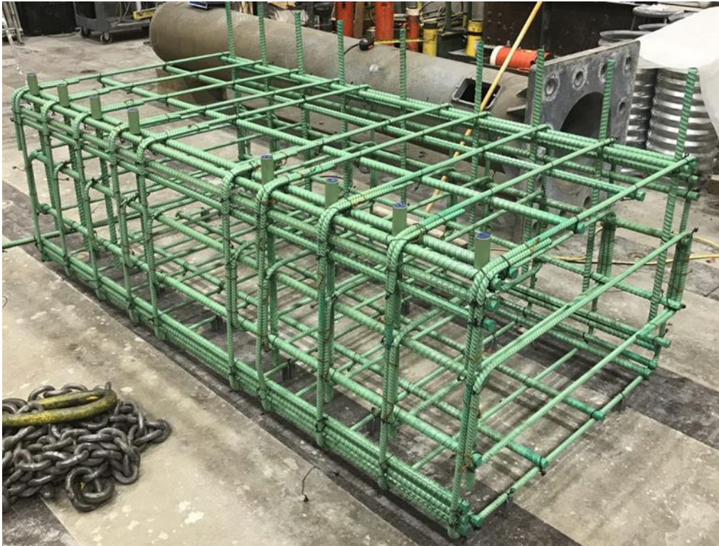
Figure 4.1 UHPC-Joint pile cap reinforcing cage.
