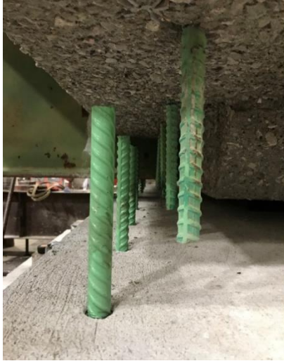
Figure 4.19 Front connection bars with installed threaded bars in pile cap.
