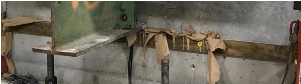
Figure 4.62 Pile coupler grout bed completed.
