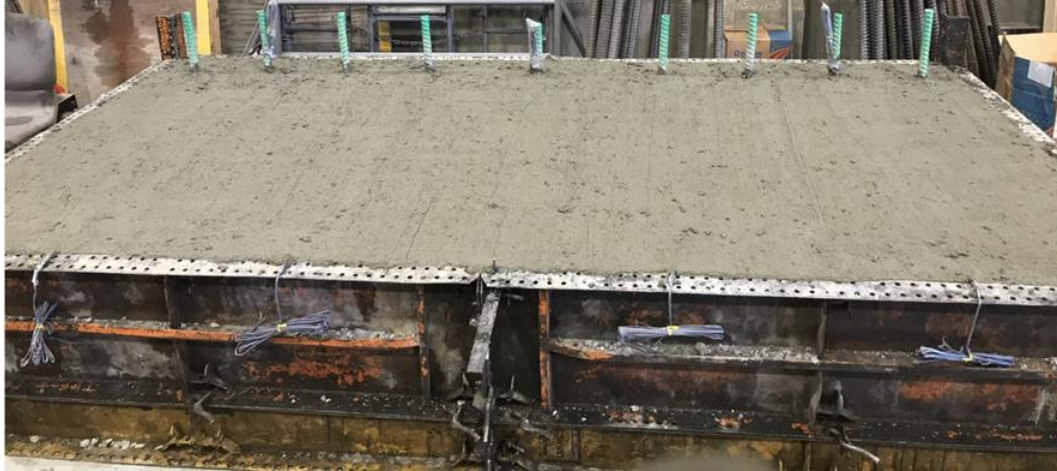
Figure 4.3 UHPC-Joint pile cap cast in concrete.
