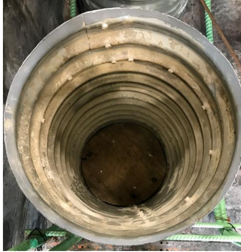
Figure 4.46 Plywood alignment of integral diaphragm CMP.
