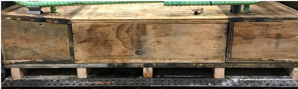
Figure 4.9 UHPC integral diaphragm bottom formwork side view.
