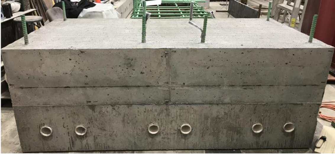
Figure 4.26 GRBC pile cap completed.
