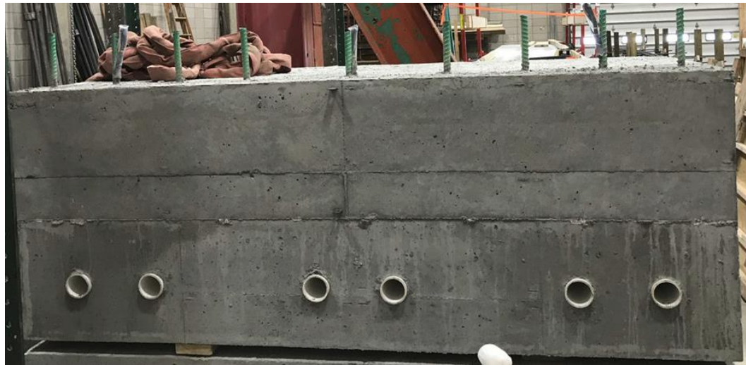
Figure 4.4 UHPC-Joint pile cap completed.
