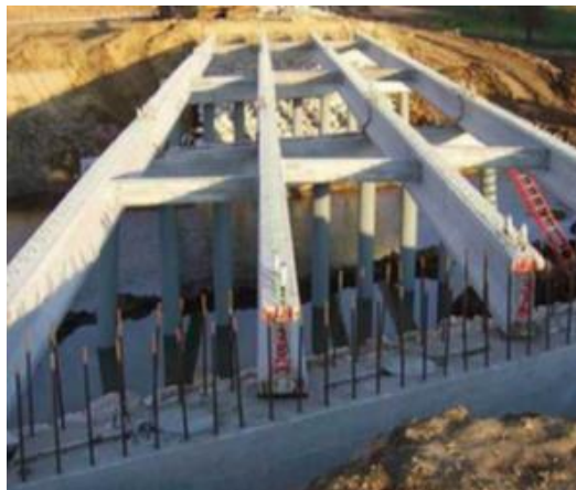
Figure 2.24 Bridge girders in final locations. (Wipf, Klaiber, & Hockerman, 2009)
