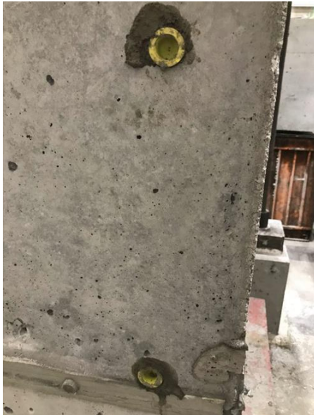
Figure 4.38 GRBC grout sleeve completed.
