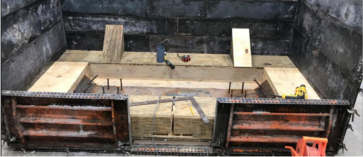
Figure 4.8 UHPC integral diaphragm formwork completed.
