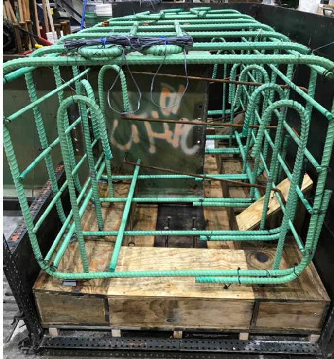
Figure 4.10 UHPC integral diaphragm reinforcement cage.
