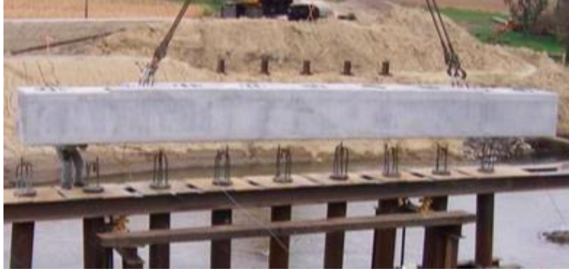
Figure 2.20 Pier cap being lowered in place. (Wipf, Klaiber, & Hockerman, 2009)
