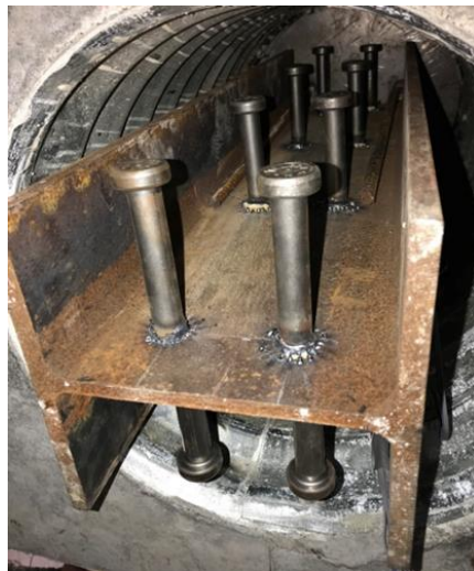
Figure 4.55 Steel section coupler with shear studs.
