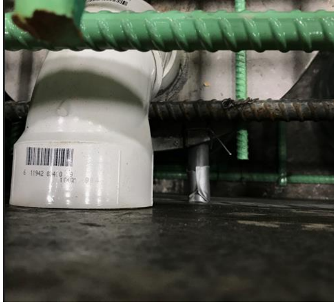
Figure 4.49 CMP ducts against formwork.
