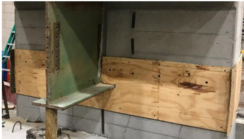
Figure 4.20 Front face joint formwork with air ports.
