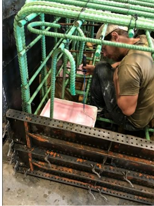
Figure 4.13 Form retarder being applied to integral diaphragm formwork.
