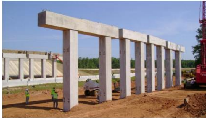
Figure 2.12 Precast open frame pier bent constructed in Georgia. (Culmo M. P., 2011)
