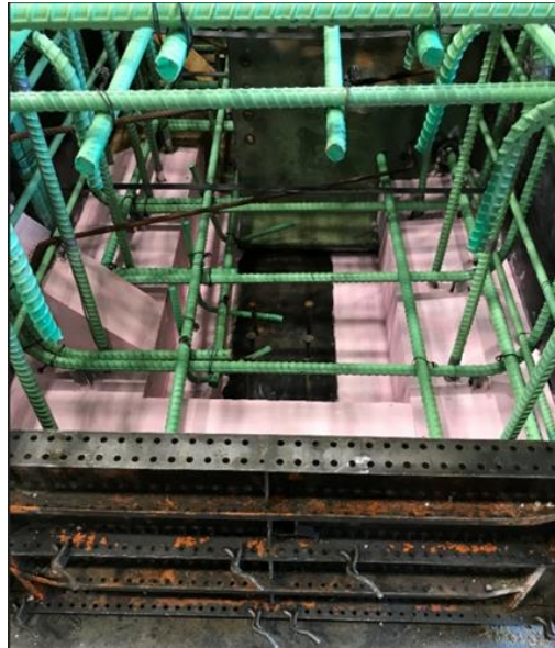
Figure 4.14 Form retarder application completed.
