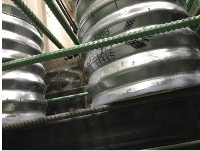
Figure 4.40 Salvage reinforcing steel bar holding up CMPs.
