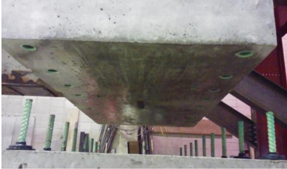
Figure 2.47 Integral diaphragm placement. (Hosteng, Phares, & Redd, 2016)
