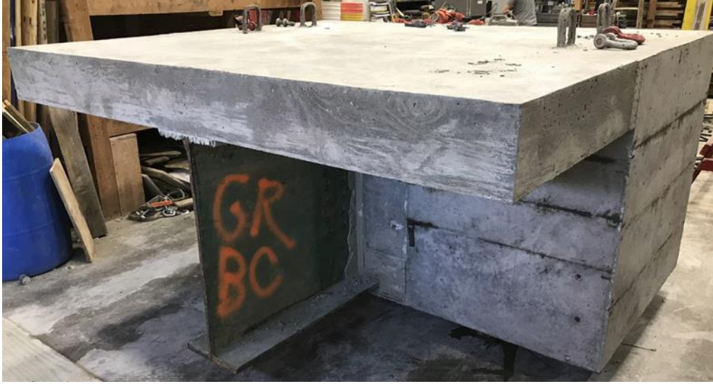
Figure 4.32 GRBC integral diaphragm completed.
