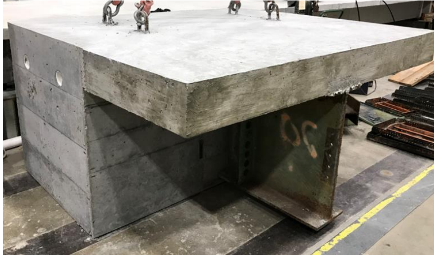
Figure 4.52 Pile coupler integral diaphragm completed.
