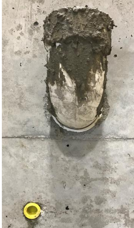
Figure 4.60 SCC completed install with 1 in. duct plugged and 3 in. duct filled.
