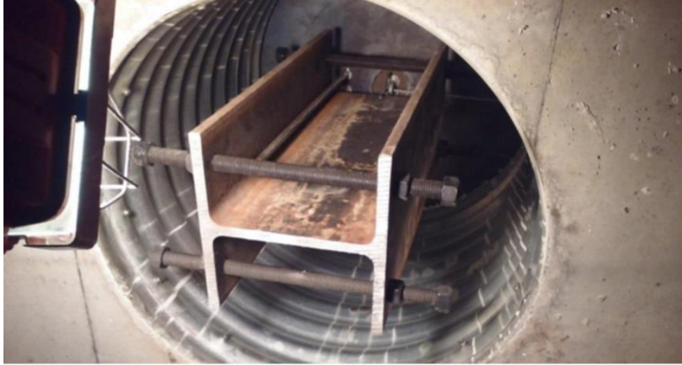
Figure 2.49 Suspended HP sections. (Hosteng, Phares, & Redd, 2016)
