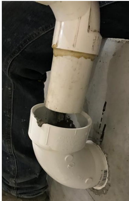
Figure 4.59 SCC installed through 3 in. duct.
