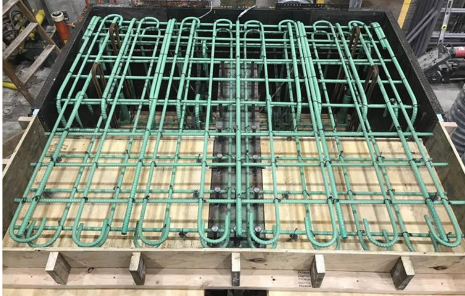
Figure 4.30 GRBC reinforcing cage.
