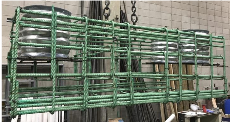
Figure 4.39 Pile coupler pile cap reinforcing cage.
