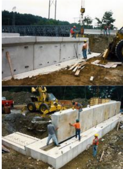
Figure 2.36 Precast abutment wall and footings with grouted coupler connections in Massachusetts. (Kapur, et al., 2012)
