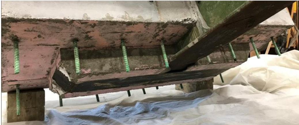
Figure 4.16 UHPC integral diaphragm completed.
