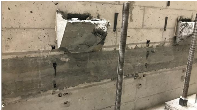
Figure 5.15 UHPC joint rear face after testing.
