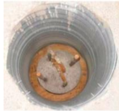
Figure 2.21 Pier cap final location (left) Pipe pile in CMP void (right). (Wipf, Klaiber, & Hockerman, 2009)
