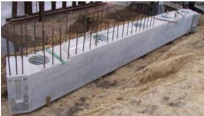
Figure 2.19 Abutment cap final position (left) H-pile in CMP void (right). (Wipf, Klaiber, & Hockerman, 2009)
