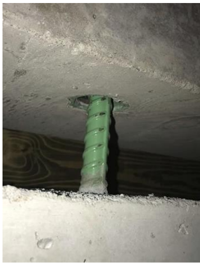
Figure 4.34 GRBC connection alignment.
