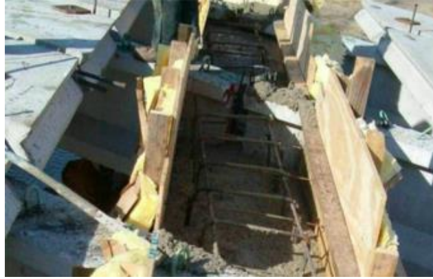
Figure 2.25 Pier cap diaphragm formwork for beam ends. (Wipf, Klaiber, & Hockerman, 2009)
