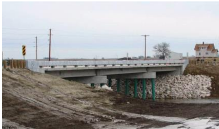
Figure 2.27 Completed bridge. (Wipf, Klaiber, & Hockerman, 2009)
