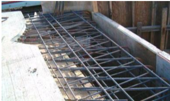
Figure 2.26 Abutment cap diaphragm formwork for beam ends. (Wipf, Klaiber, & Hockerman, 2009)
