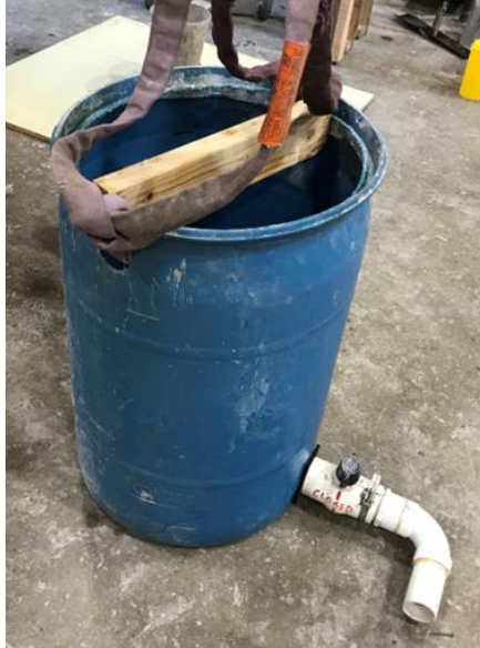
Figure 4.58 Barrel with funnel to install SCC.
