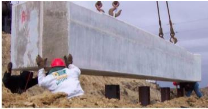
Figure 2.18 Abutment cap being lowered in place. (Wipf, Klaiber, & Hockerman, 2009)
