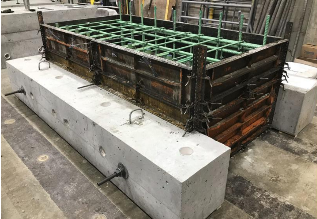
Figure 4.2 UHPC-Joint pile cap formwork.
